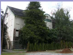
Lonsdale School is scheduled for demolition
